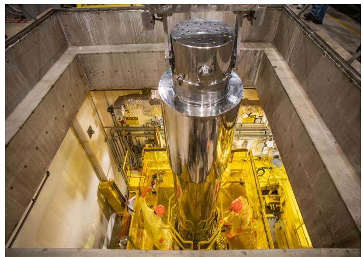
TEF personnel receive rods shipped from the Tennessee Valley Authority in preparation for extracting tritium for the nation’s nuclear deterrent
